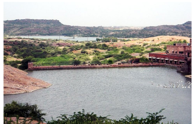
Fig. 9 Bijolai palace hydro-geosite with rhyolite hills and Kayalana Lake in background
